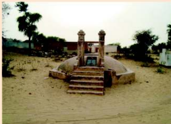
Tanka in a village used for storing water/rainwater
